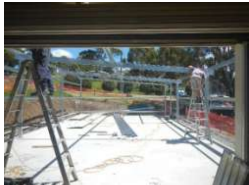
Work re-commenced 16 th December
